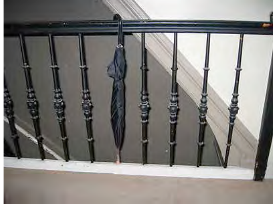
Staircase Repair, made by someone who participated with the competition.
