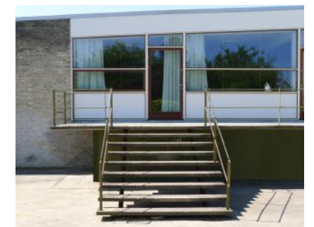
Udskolingsbygning østfacade East facade of secondary education building
