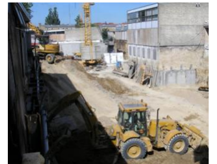
Byggeri, skolegården bortgravet Construction, school playground dug up
