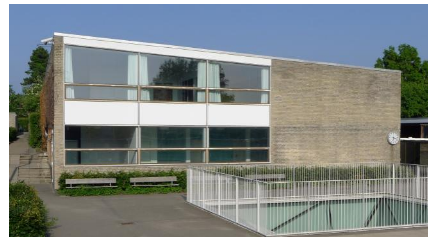
Udskolingsbygning vestfacade West facade of secondary education building
